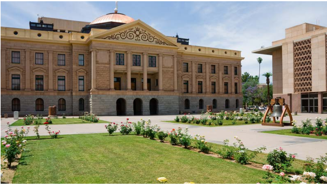
State Capitol Building - Phoenix Arizona
