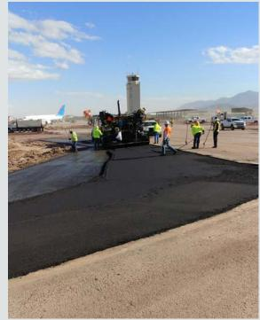
feet wide with gravel shoulders. The entire width of the pavement will be rehabilitated by milling 2 inches to remove the porous friction course (PFC) (P–402) and paving back 3 inches (P–401), for a distance of 7,150 feet. This effort will bring the strength of the finished structural section up to a minimum Pavement Condition Index (PCI) of 67. (con't)
