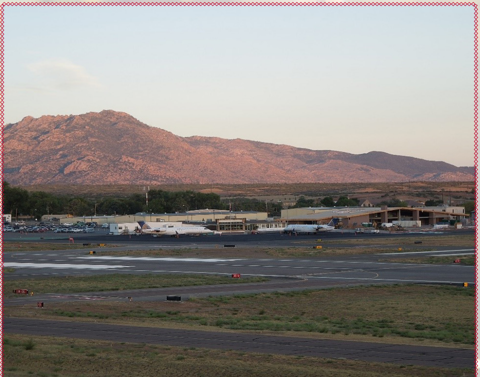
New Passenger Terminal Under Construction at PRC
